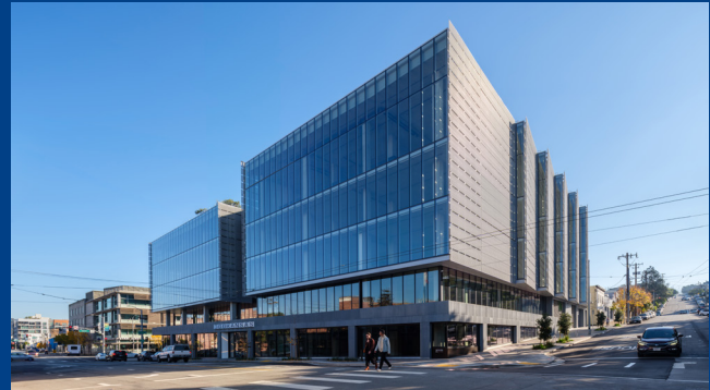
Figure 6. North and west facades of Potrero Hill Innovation Center, showing sawtooth bay windows on the west.
