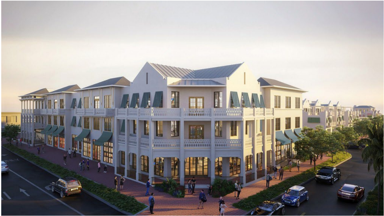
Sundy Village office & retail. Rendering of the three-story office and retail building. Image courtesy of Pebb Capital.
