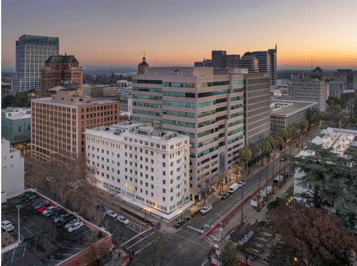
The Saint Clare at Capitol Park exterior. Image courtesy of Page & Turnbull
