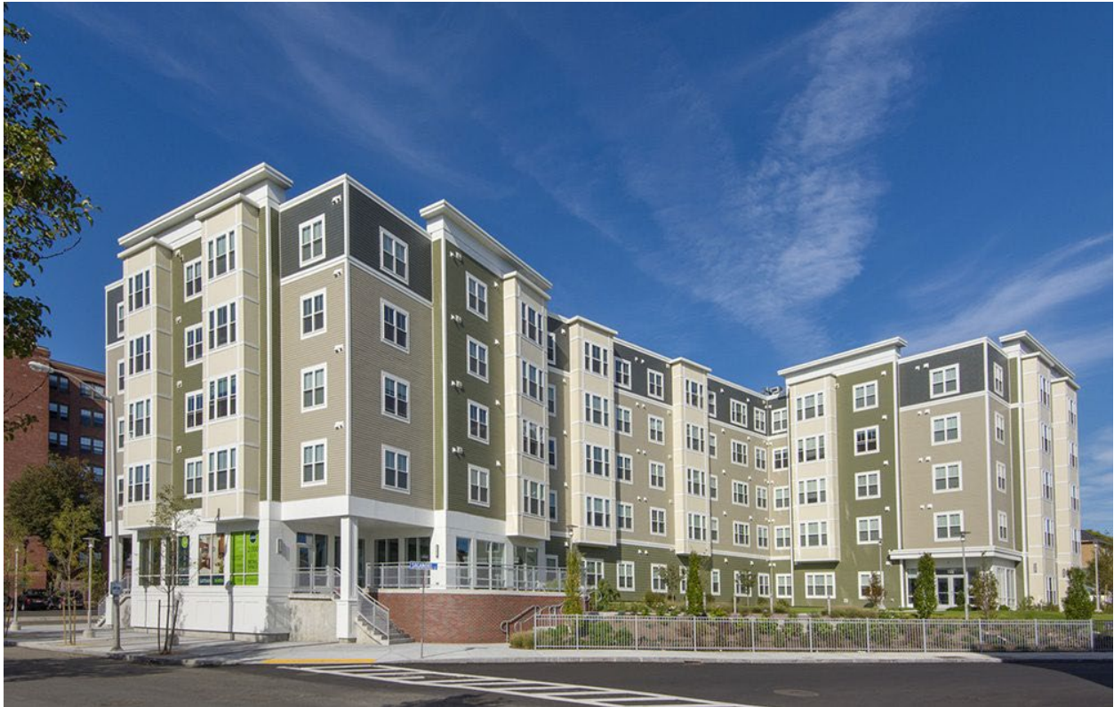
Gateway North Apartments in Lynn, Mass., features 71 units for mixed incomes.
