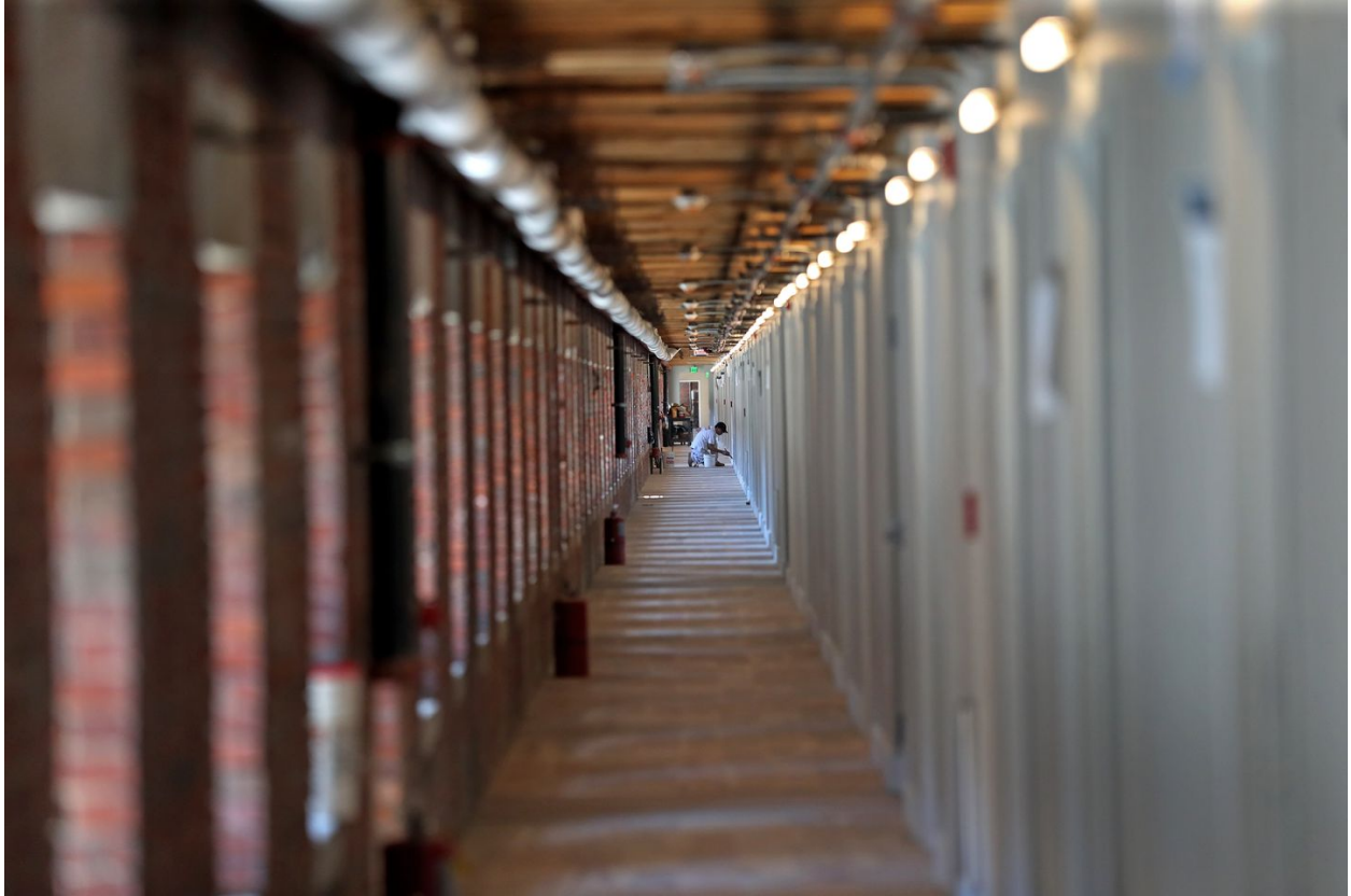
A painter does some finish work along the long hallways that once were used for making rope. DAVID L. RYAN/GLOBE STAFF
