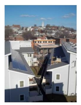
Green features are incorporated throughout the plan and architecture, says Jay Szymanski, AIA, project architect and associate at The Architectural Team. "The buildings are oriented to maximize solar exposure, with carefully designed exterior envelopes that inherently reduce heating and cooling loads," says Szymanski. "Efficient mechanical systems, appliances and lighting are matched by new policies at Old Colony to limit waste and improve indoor air quality."
